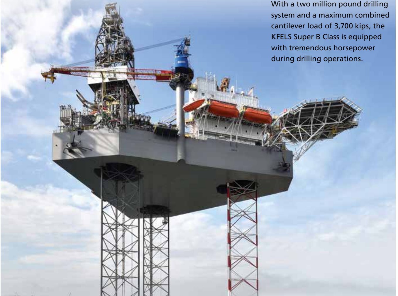
Keppel continues to deliver rigs that provide superior performance and are efficient and reliable
