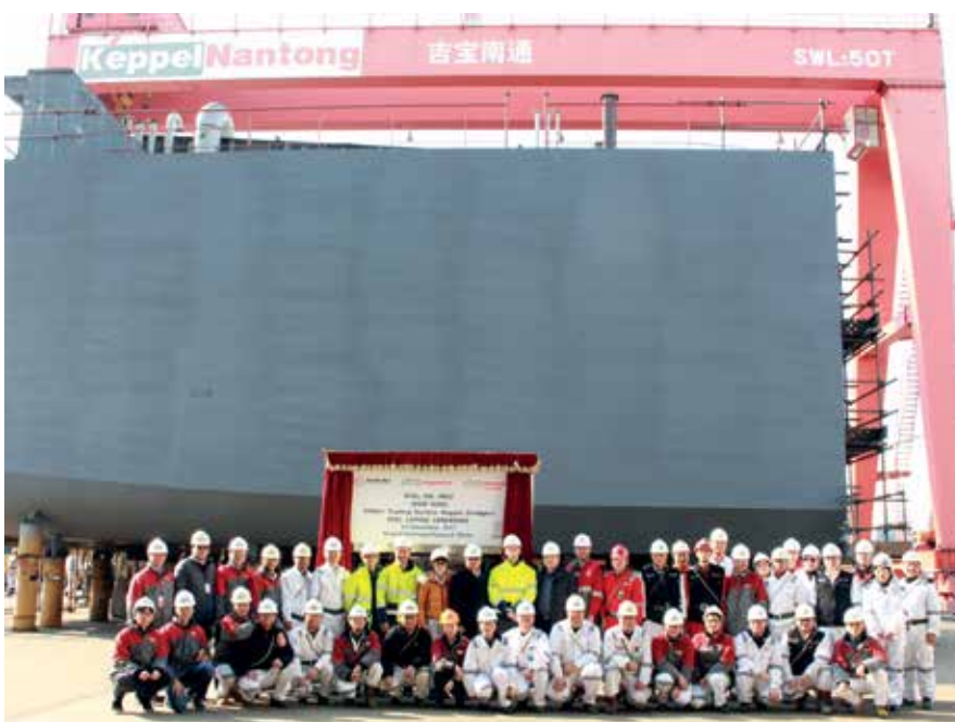
The successful keel laying for the third TSHD for the Jan De Nul Group marked another milestone in Keppel Singmarine's track record for non-oil and gas solutions
